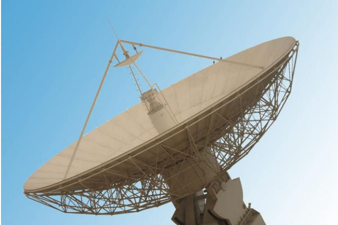
Really large antennas
